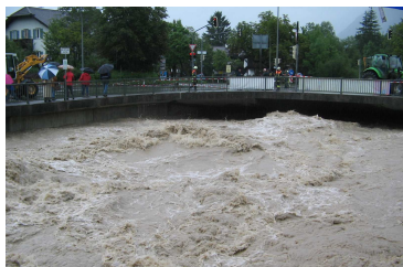
Loisachbrücke in GAP:
